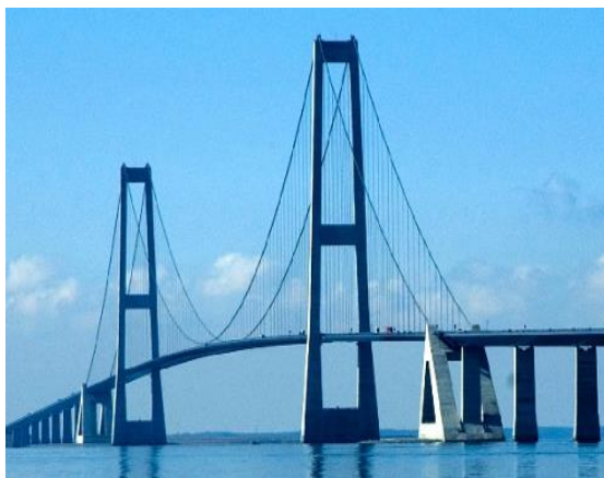
Fig. 6: Great Belt Suspension Bridge
